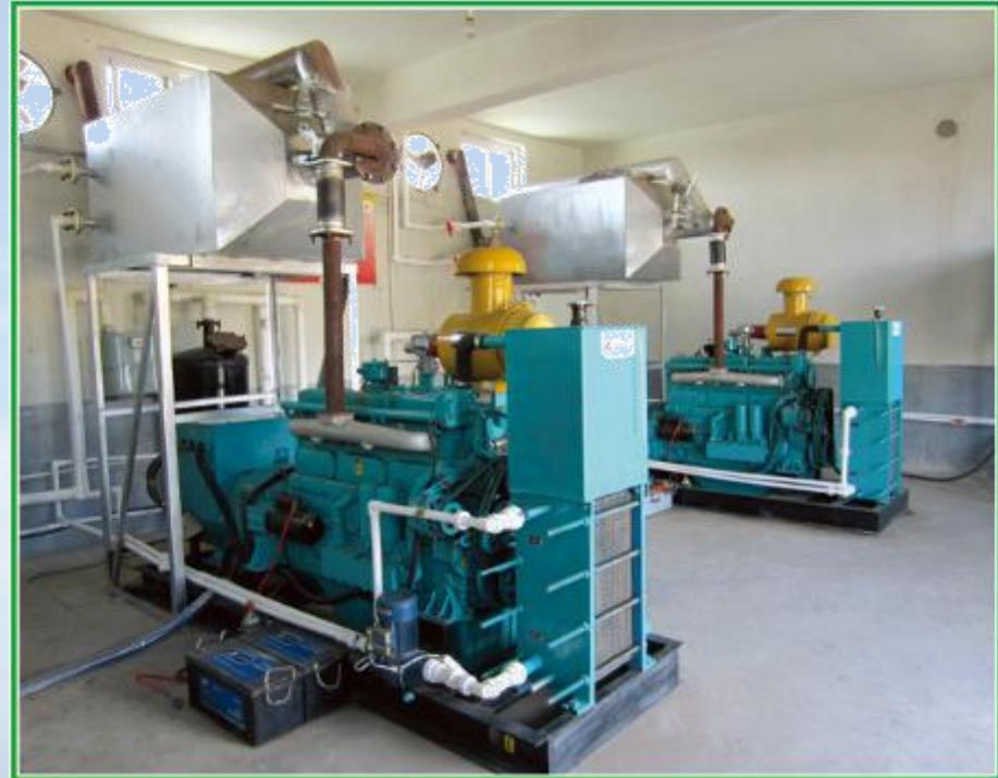
This series gas generator set fully exchanged the heat of exhaust gas and high temperature circulating water of the engine through gas heat recovery system and plate heat exchanger in order to achieve the purpose of energy-utilized.
