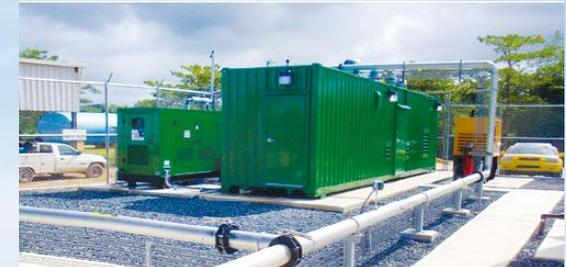
200kW, Biogas generator, Puerto Rico
