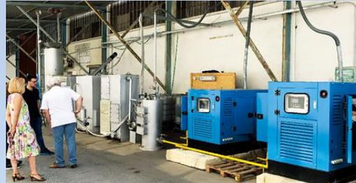
50kW, Gasification system, MARCON Italy
