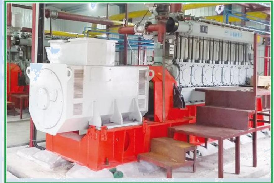
The biomass gas generator using the syngas produced from gasification system on waster rice husk, straw, wood flour, wood chips as raw materials.
